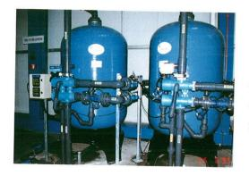
Filtration plant for a pharmaceutical company. The company was observing stains during steam sterilisation on their rubber products. After installation of the filtration plant, the stains disappeared. The plant operation is completely automatic.
