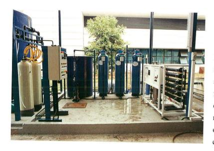
Pure water treatment plant for a surface coating company. The scheme incorporates media filter, carbon filter, base exchanger, reverse osmosis and mixed bed columns. The operation of the plant is completely automatic.
